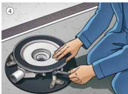
4 Position the drain and sound insulating mat and, and adjust it to exactly the right height, with help from the height-adjustable assembly feet.
