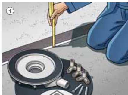
1 Measure the floor construction height, here: 85 mm.
