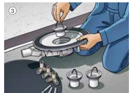
3 Choose one of the immersion pipes included in the scope of delivery, here: using the shortest model.
